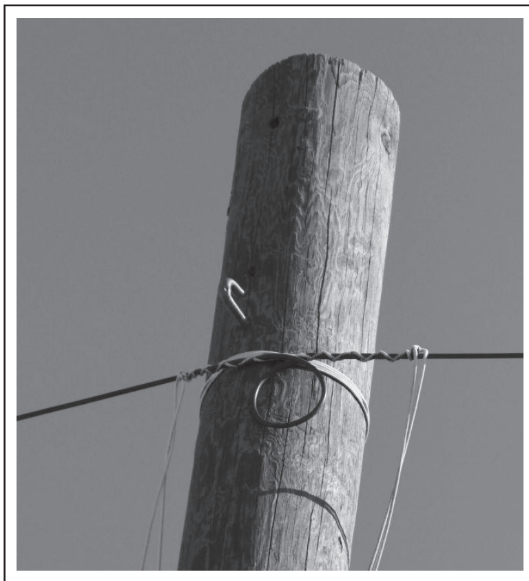
Figure 3-19. Drip loop
