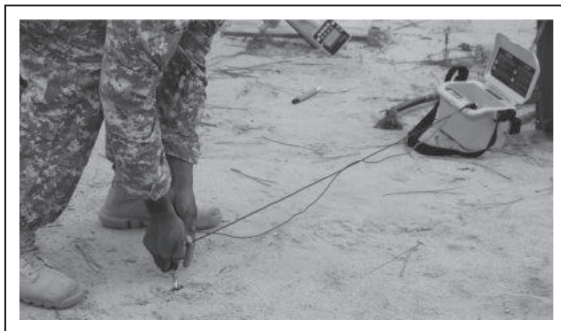
Figure 3-29. Direct connect ground rod connection
